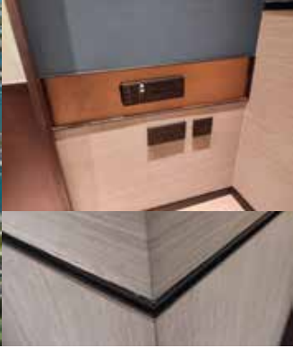
Project: Rosewood Doha Client: SECC Work: Metal Works
