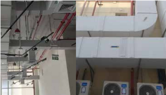
Project: Car Show Room, Pearl Client: DIFM Work: HVAC Works
